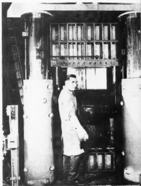
Lower part of the first 4000-lb block, like one above, cracked under stress before mold's assembly.
